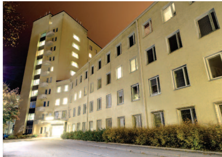
South Karelia Central Hospital in Lappeenranta, Finland.
